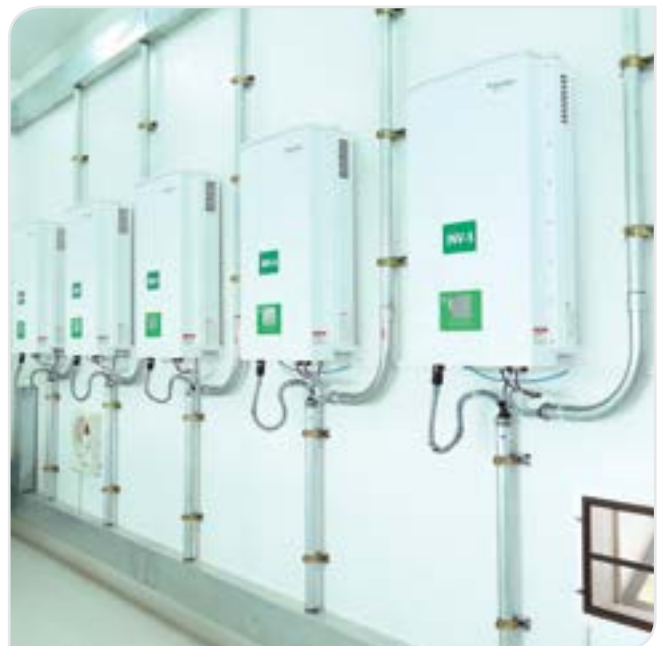
Phetchabun, Thailand PV power plant 3.3 MW
