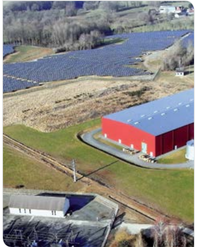
Bonnat, France PV power plant 5.4 MW
