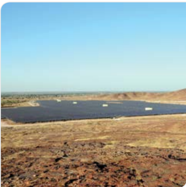
Osiyan, India PV power plant 5 MW
