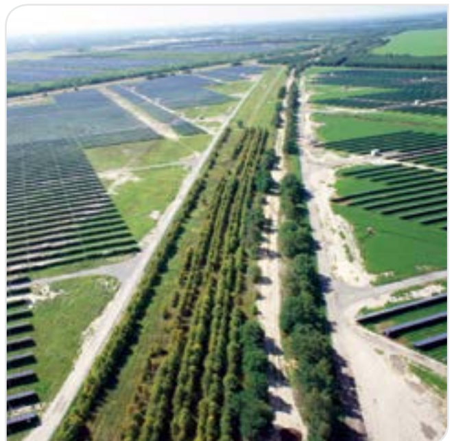
Senftenberg, Germany PV power plant 82 MW
